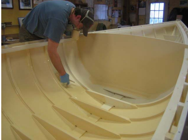
Fig. 20) MURMUR interior paint looking forward
