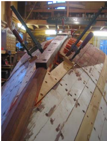
Fig. 17) Laminated mahogany stem & plank keel
