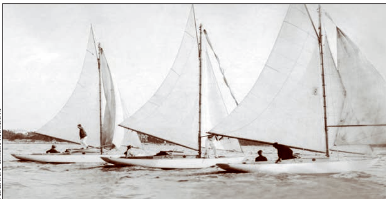
In 1925, the original Manchester 17½-footers (left) had their sail plans altered from gaff to Marconi rig (right).
